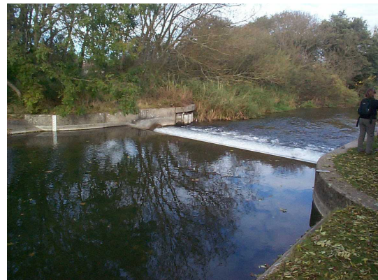
River Lambourn at Shaw weir
